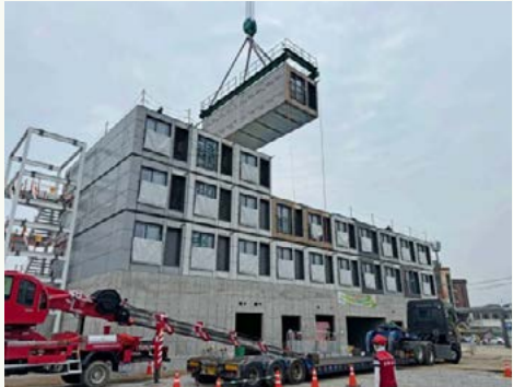
Module Lifting and Installation
