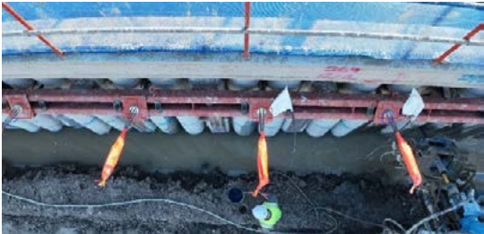
AI-Based Safety Inspection for Temporary Structures
