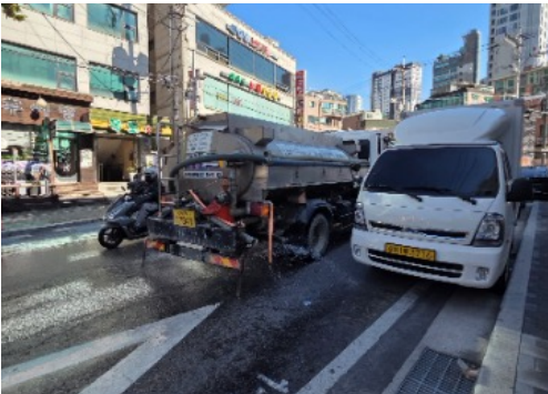
Spraying Water on Surrounding Roads to Prevent Fugitive Dust at Mapo Xi
